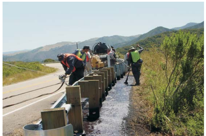
Two crews are simultaneously applying the seamless composite weed barrier on both sides of the guardrail.
