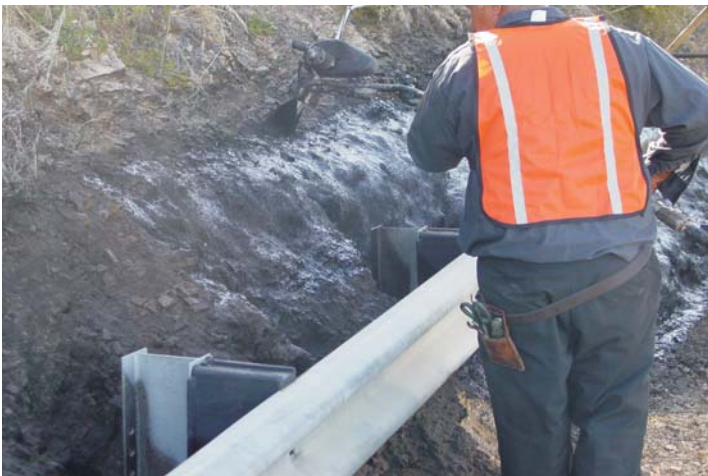
Photo of application of Seamless Composite, applied at a rate of 1.61 gallons of emulsion and .86 pounds of fiberglass reinforcement per square meter.
