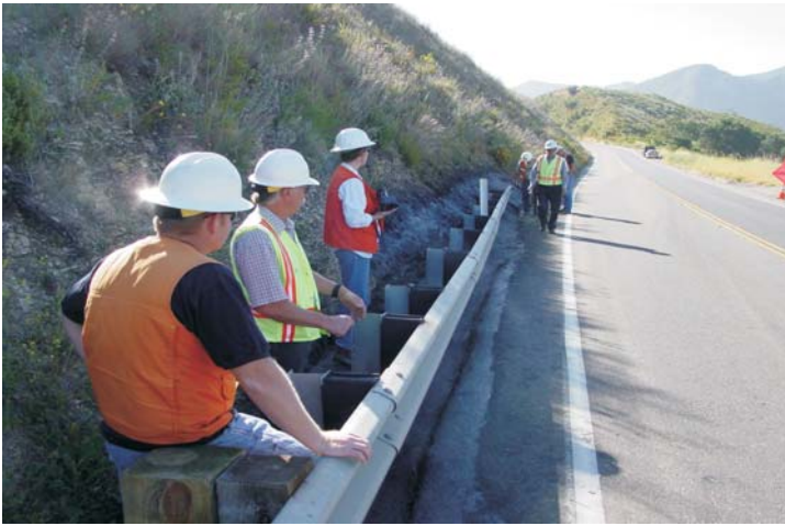
District 5 Cal Trans personnel inspect installation along side bridge abutment.
