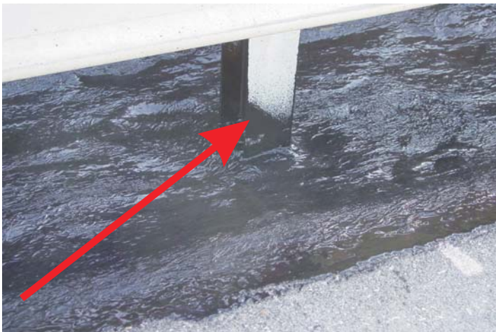
Composite is also flashed to all surfaces around guard rail posts to ensure an air and water tight seal.
