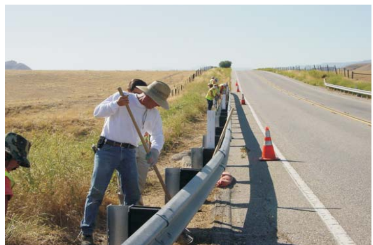
On the eastern edge of the project, CW Construction is cleaning, grubbing and compacting the soil in preparation for the spray crews.
