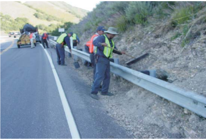
The WeatherWeld crew is cleaning out loose gravel and compacting the surface prior to their installation of the seamless composite Weed Barrier E.
