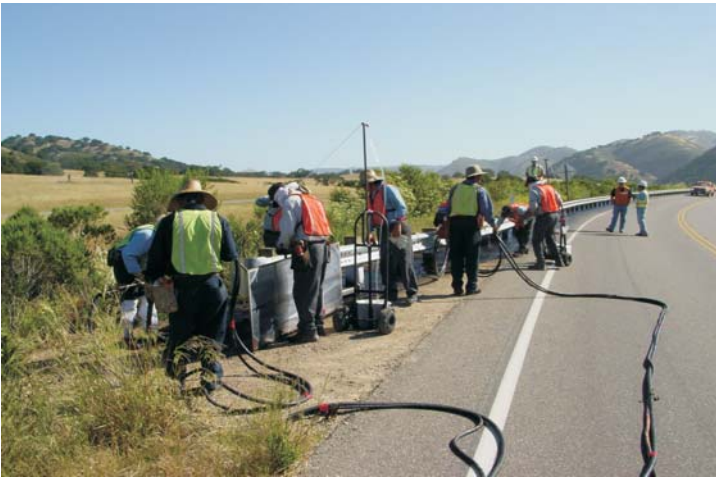
Work continues on Weed Barrier E installation as Cal Trans personnel observe.
