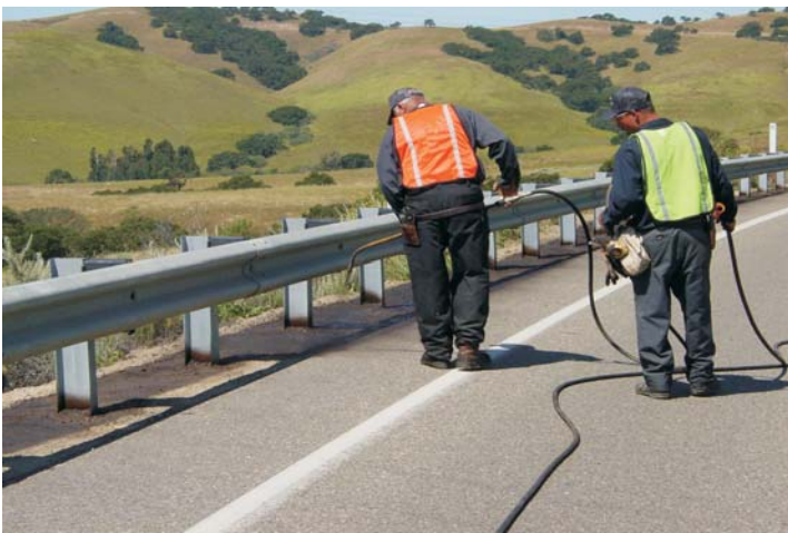
A 3:1 tack coat of water/emulsion is applied on the prepared soil surface.
