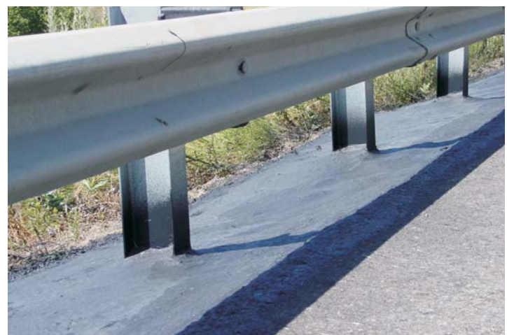
Seamless composite materials can be seen fully attached from AC roadbed lift, flashed around the guardrail supports, to the backside drip edge.
